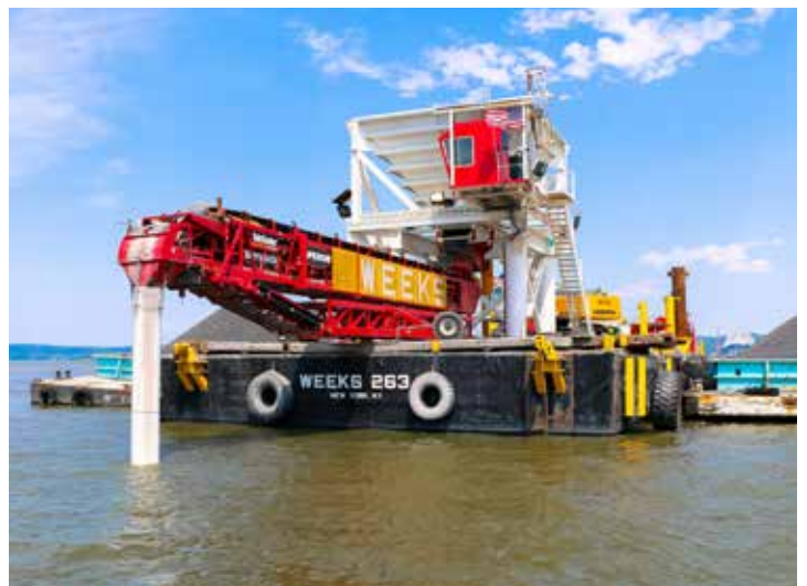
BARGE UNLOADING / DREDGE CAPPING
