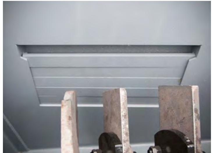
ADJUSTABLE OVERFLOW GATE
