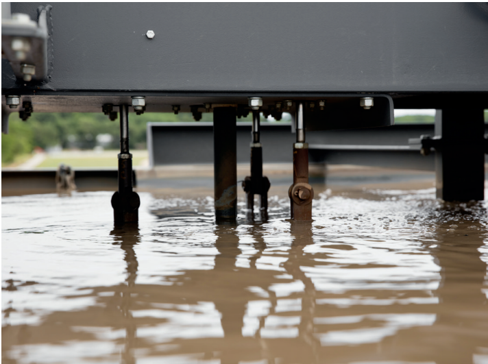
06/ FULL-LENGTH VALVE BRIDGE
